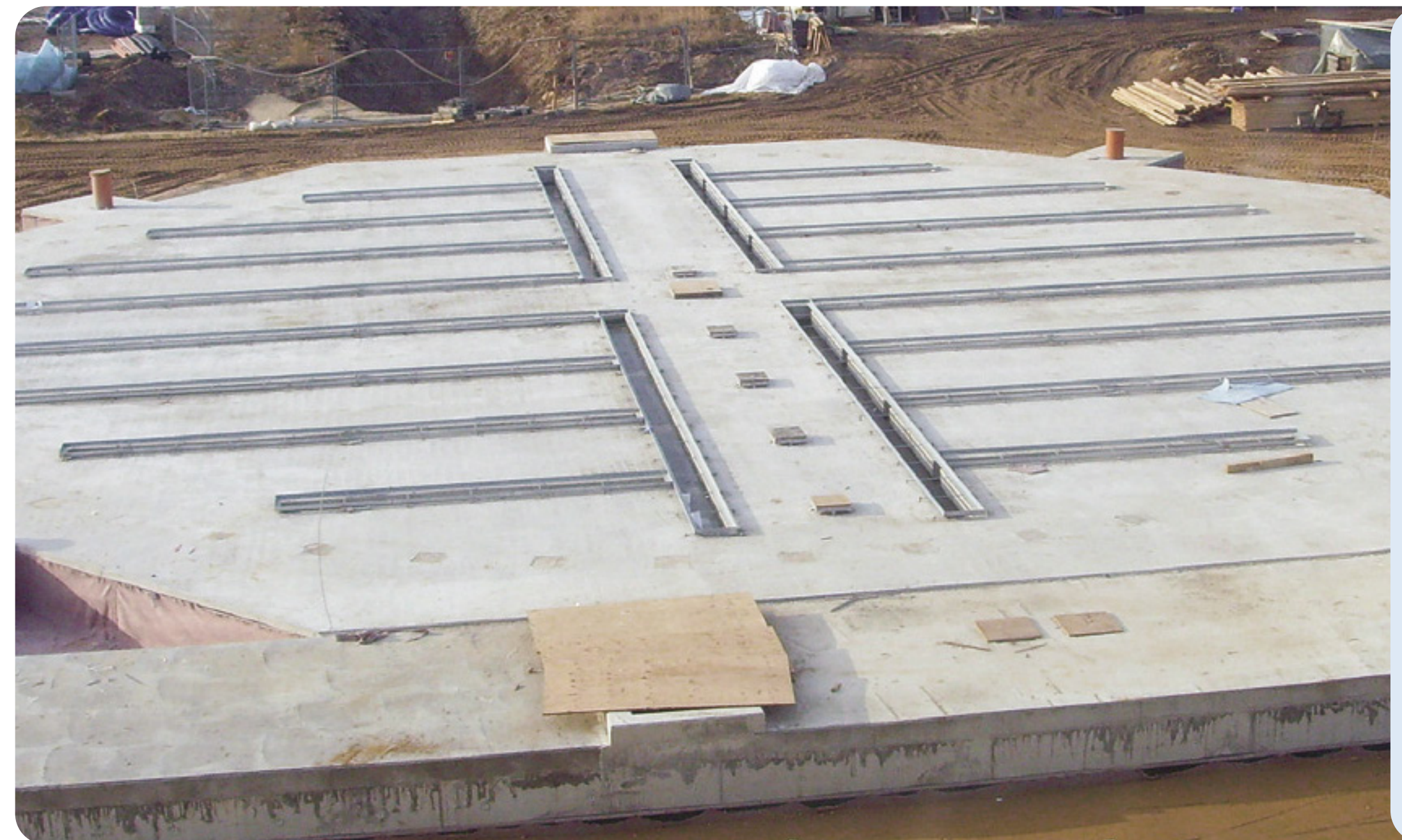
Ventilation Channels
